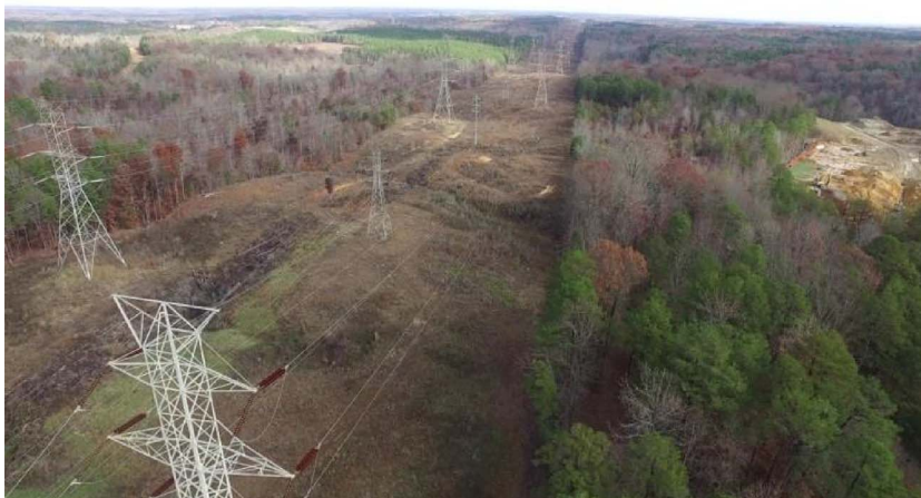
Fig. 3. Image of transmission right of way.
